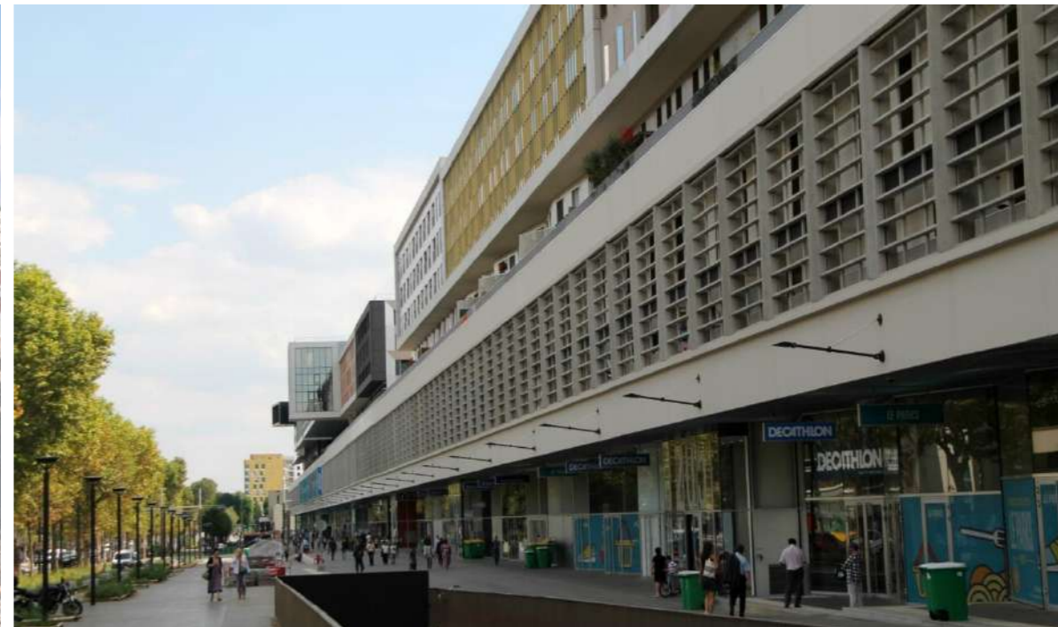
Entrepôt Macdonald – Paris – França
